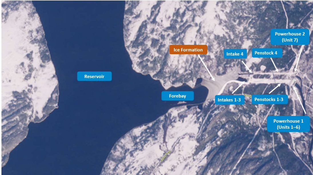
Figure 2: Satellite Imagery of Ice Formation in the BDE Forebay – January 21, 2026 4
